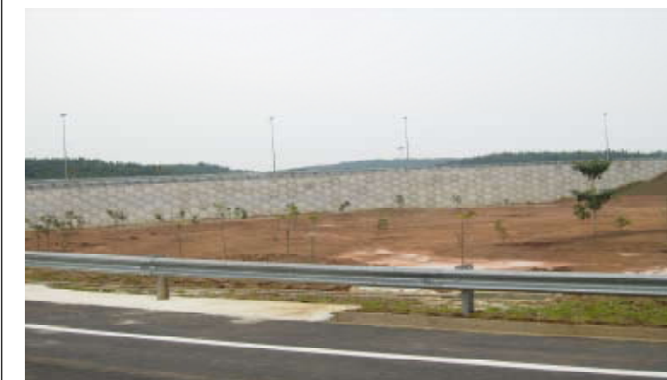
The completed Nehemiah wall at Kuantan Interchange
