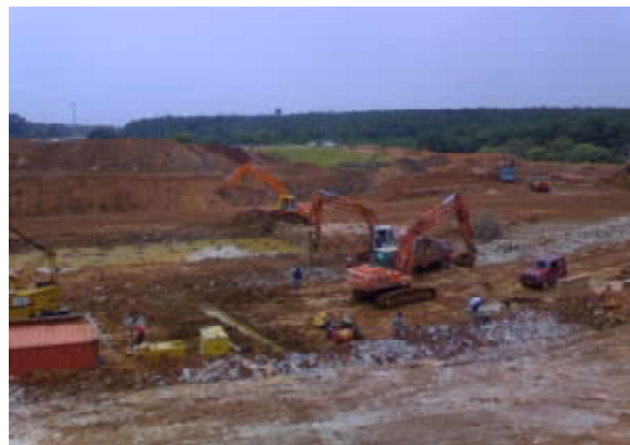
Excavation work was in progress to prepare the platform
